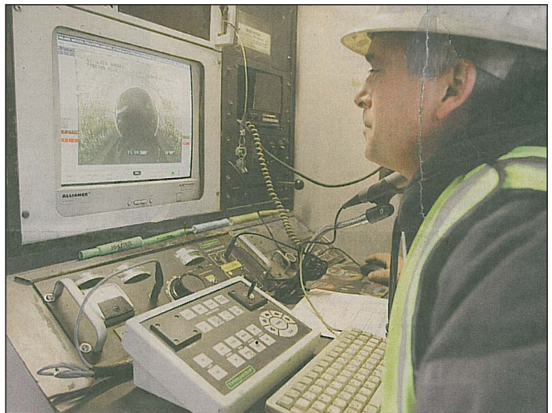
Rene Gendron operates a camera and computer to look at digital photos of underground sewer lines. A three-month project uses cameras to check St. Clair Shores sewer lines for leaking, damaged or blocked pipes.
