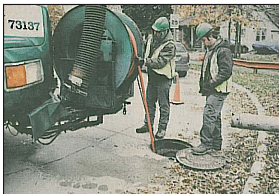
Mark LeBeau, left, and Chris McCoy pump out a sewer before a camera is put under the ground to check for problems with the pipes.
