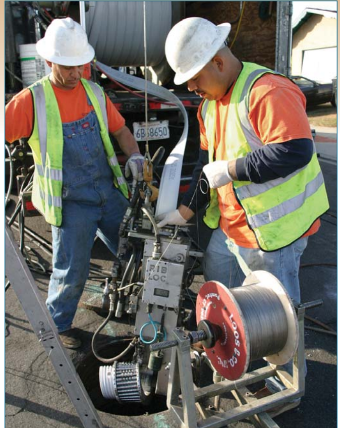
Ribloc's patented spiral winding device is small enough to fit into existing manholes.
