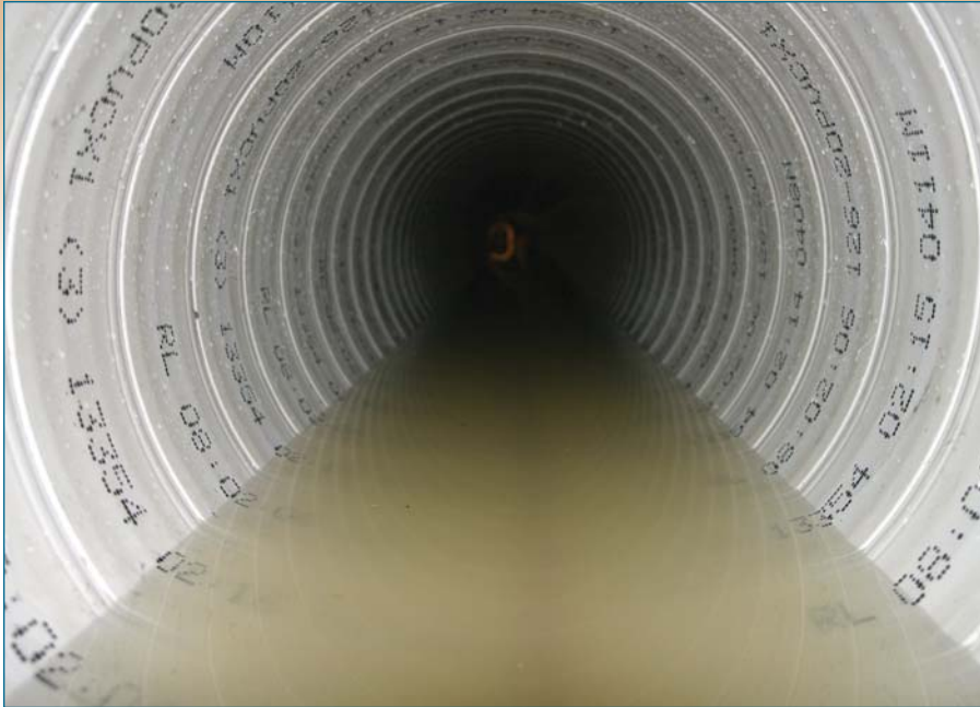
Once installed, Expanda is a continuous, tight-fitting PVC pipe from manhole to manhole.
