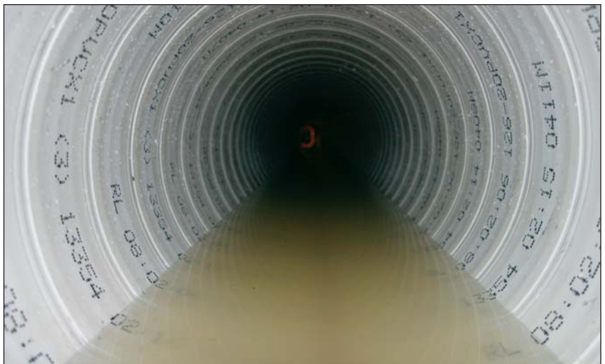
The new Expanda pipe is made of hydrogen sulfide-resistant PVC.
