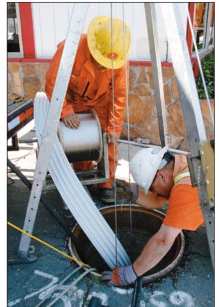
Workmen insert the Expanda profile into a manhole.
