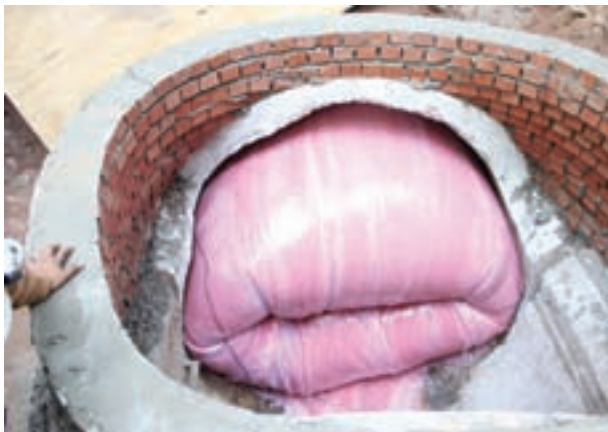
Pushing the liner through a manhole
