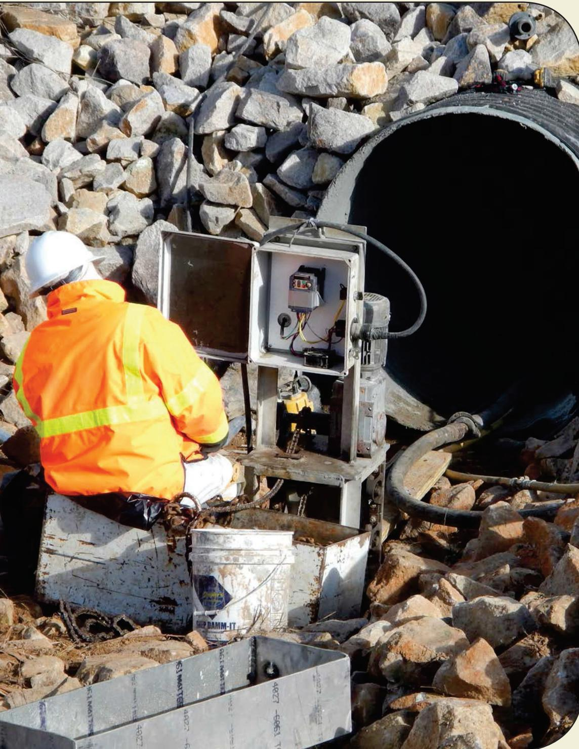
*A technician controls application of geopolymer mortar liner to rehabilitate a steel storm drainage culvert at Simmons Army Airfield, North Carolina. (U.S. Army Photo)*
