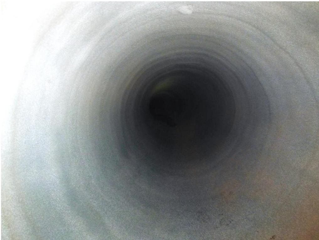
**Figure 6. Post-Lining Inspection of Lined Pipe**
