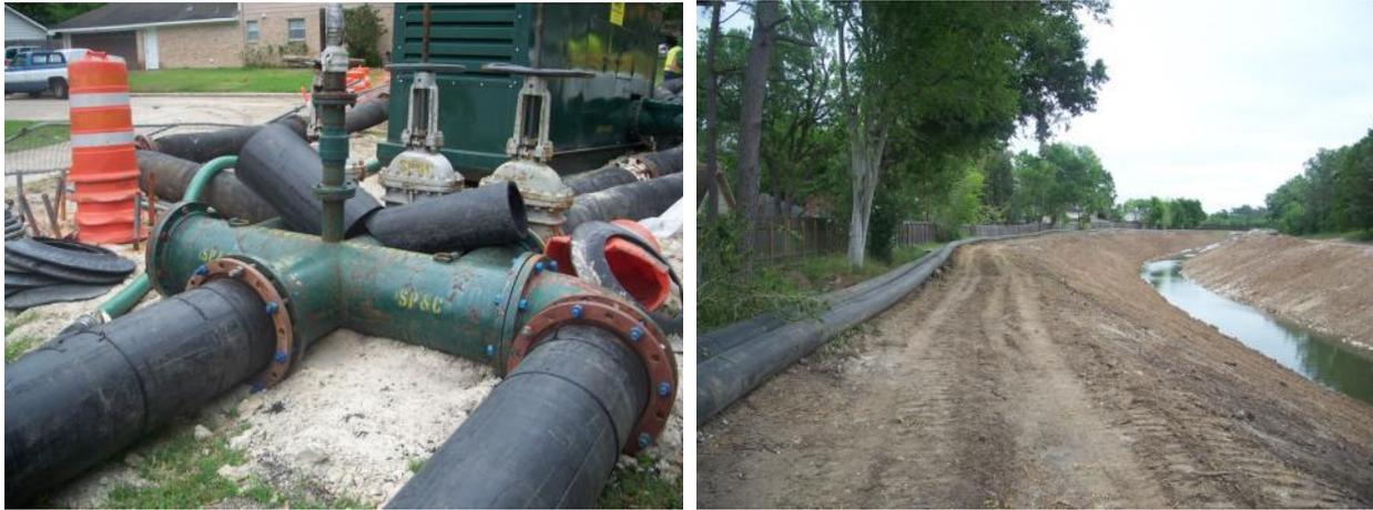
**Figure 2. Three Pipe Bypass Pipe Converging to Two (left) and Laying Parallel to an Open Channel**
