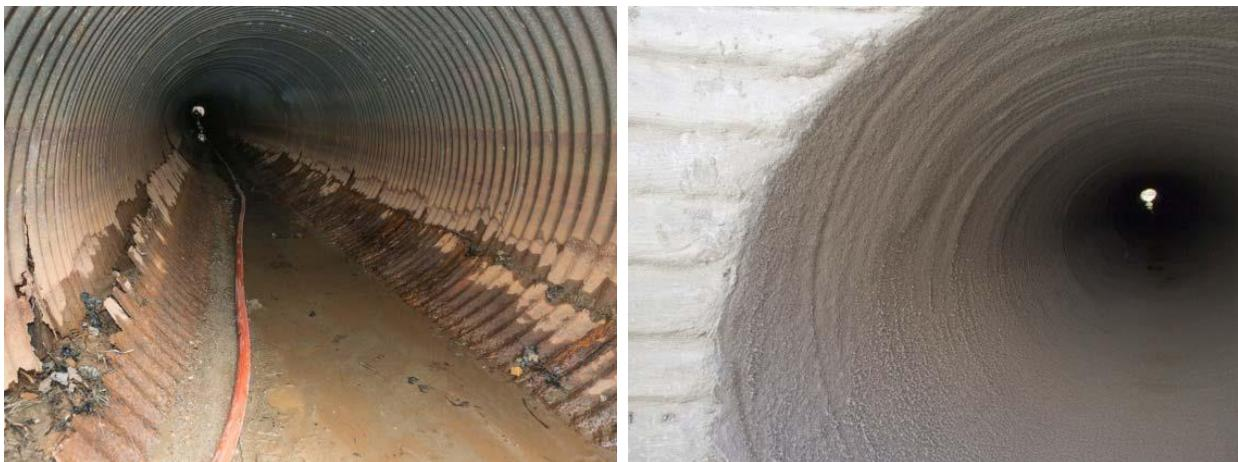
**Figure 1. Corrugated Metal Pipe Before (left) and After (right) being Rehabilitated with GeoSpray™**
